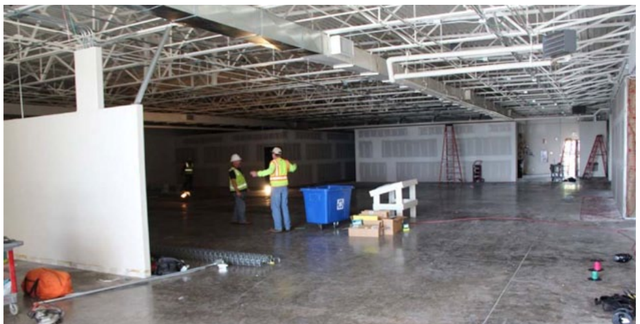
Work begins on MI Museum Project, September 2014.
